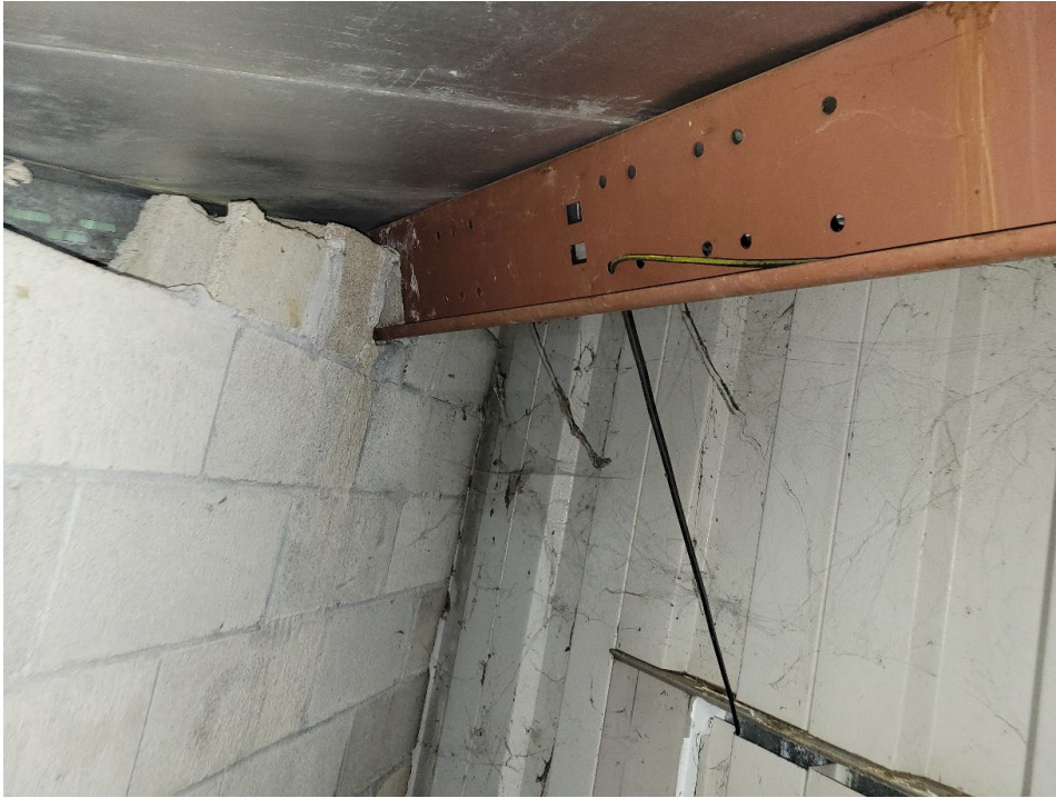
Figure 3 – Bearing of Purlins at CMU wall above Locker Room D
