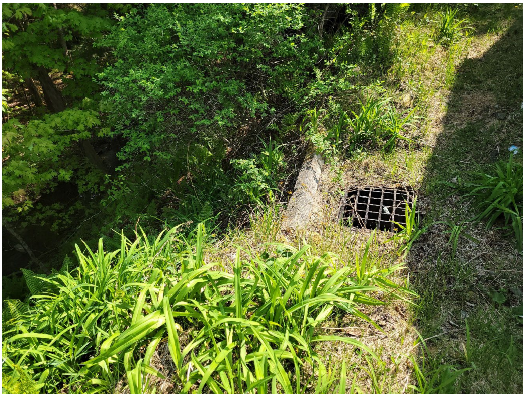
Figure 7- Steep embankment along south and west around exterior
