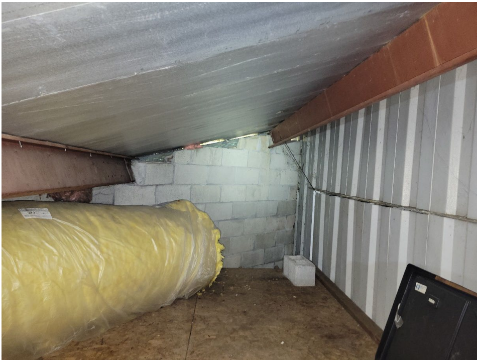
Figure 4 – Bearing of Purlins at CMU wall above Locker Room D
