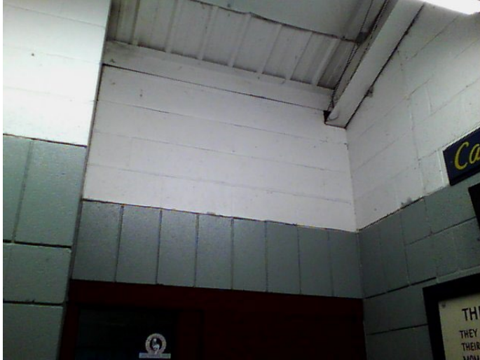
A section of this CMU wall, looking from the arena side.
